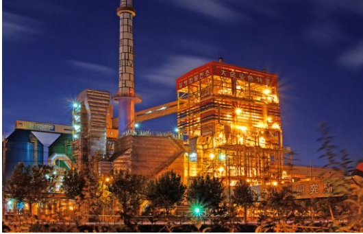
Fig. 2: Daegu combined cycle gas turbine plant.
