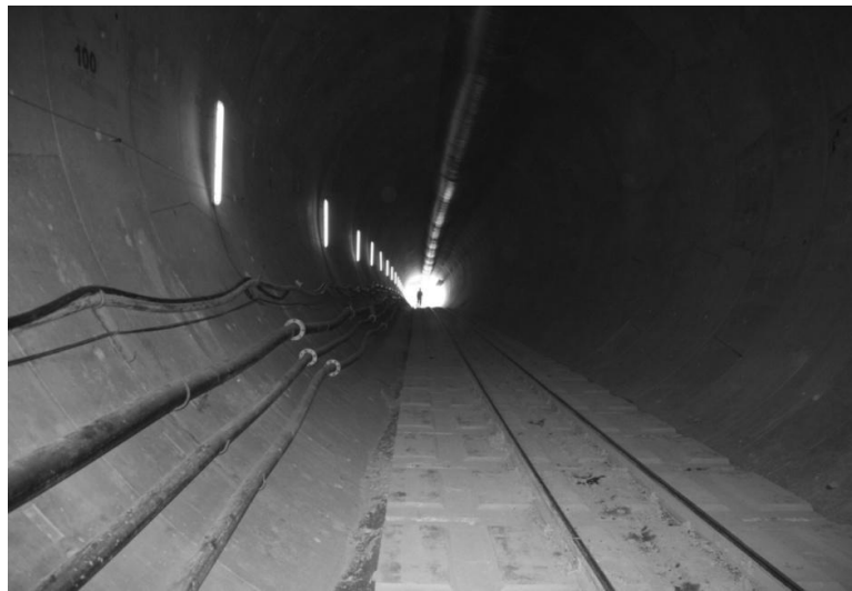
Fig. 2: View tunnels and water pipes.
